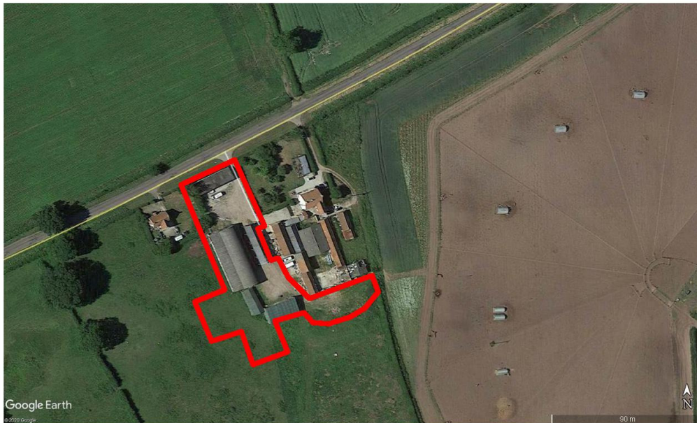
Figure 1. Google Earth aerial view of site
